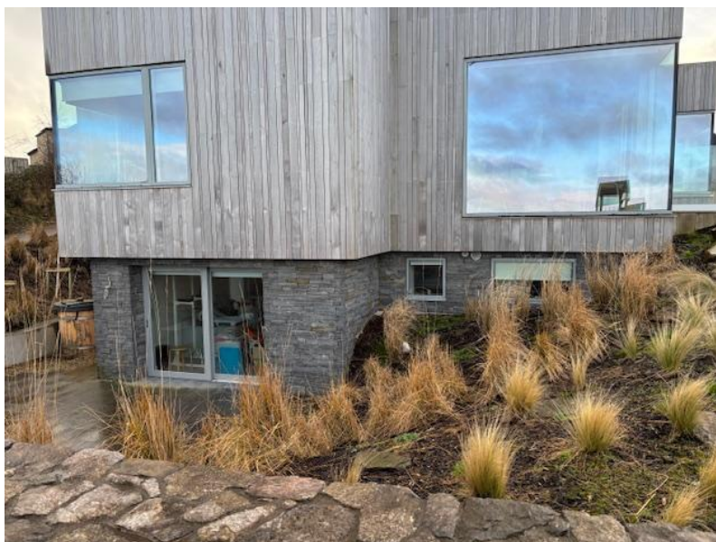
04 Stone Cladding on Basement Level
