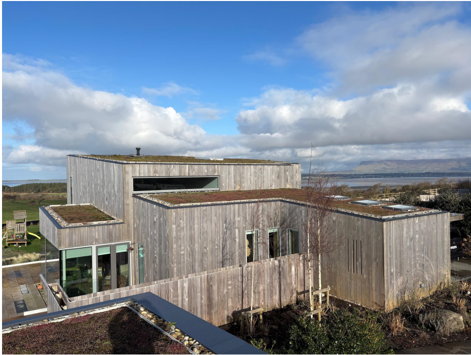
02 View showing Sedum roof on garage and house
